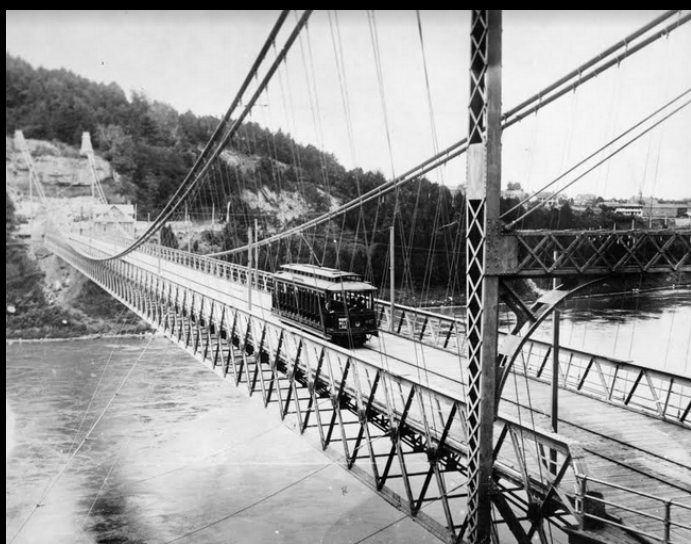
THE LOWER SUSPENSION BRIDGE – Built in 1889 by the International Railway Company, the bridge connected Lewiston NY and Queenston Ontario.
